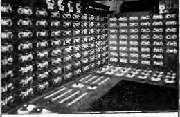
Lighting equipment installed at the new Chicago Givic Opera House, Chicago. Left, Thyratron rack. Above, lighting-director's control board. Right, reactor and disconnecting-switch rack.
